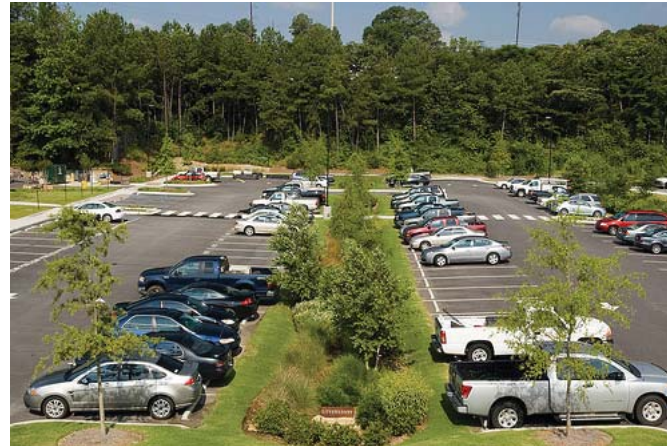
Stormwater island in parking lot
