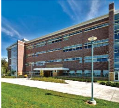
Main entrance defined by architecture
