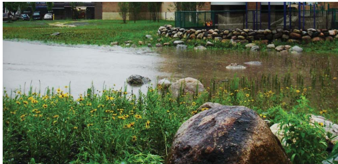
Rain garden detention with native plant material
