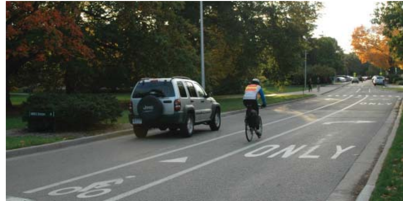
Delineated bike lanes on the Michigan State University Campus (image courtesy of MSU Bikes)
