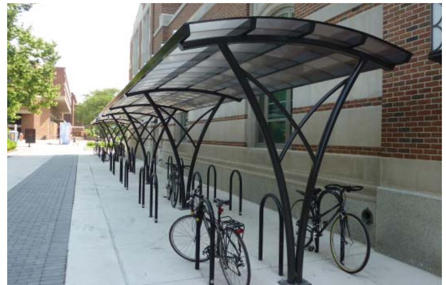
Weather protected exterior bike parking
